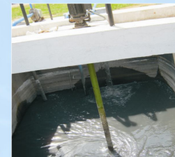
Equilisation Tank Agitator
