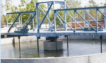
Rotating Bridge - Peripheral Drive
