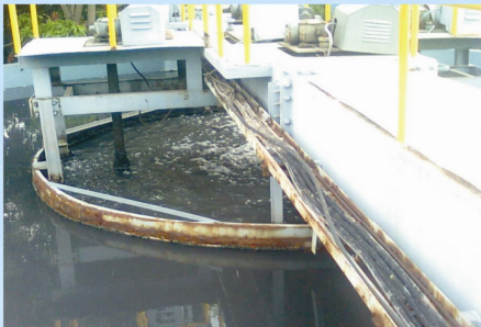
"HRSCC - Centrally Driven With Dual Stack Concentric Mixer Drive".
