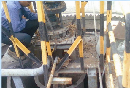
"HRSCC - Centrally Driven With Dual Stack Concentric Mixer Drive".
